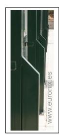
The structural system is composed of 26 support posts, each of which is resting on an individual ground socket plate and with reinforcing support plates (profiles at 1000mm height of 100x60x3mm for the posts supporting the glass closure.)
