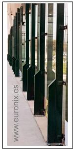
The main structure of the court is made of 100x60x2mm and 60x60x2 laminated / hot rolled steel profiles with quality S-275-JR and S-235-JR.
