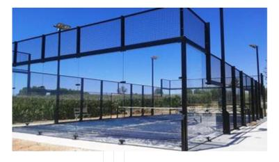
The height of the posts vary between 3,4 and 6 meters and are equipped with angle profiles and corresponding fixing plates for the she secure tightening of the surrounding closure walls composed of either tempered glass or steel framed wire mesh.
