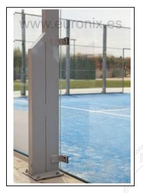
The main structure of the court is made of 120x60x3mm laminated / hot rolled steel profiles with quality S-275-JR and S-235-JR.
